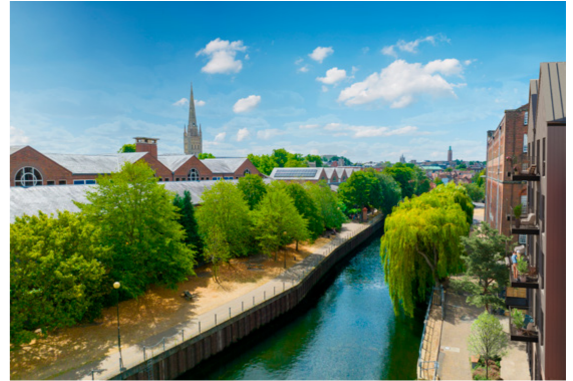
Computer generated image of the Tiernain Building at St James Quay
